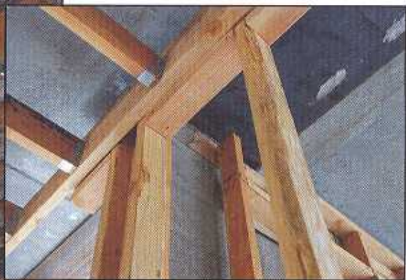
Interior non-structural wall connections.
