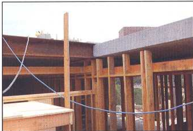
Second floor spancrete diaphragm.
