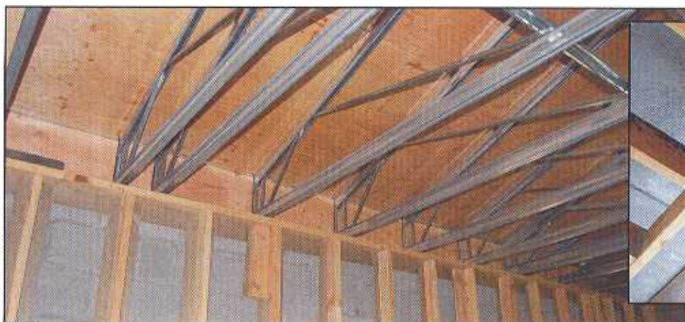
Roof Truss Diaphragm connection.
