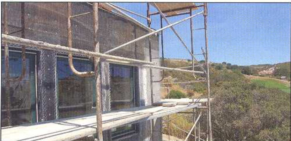
Exterior stucco application.
