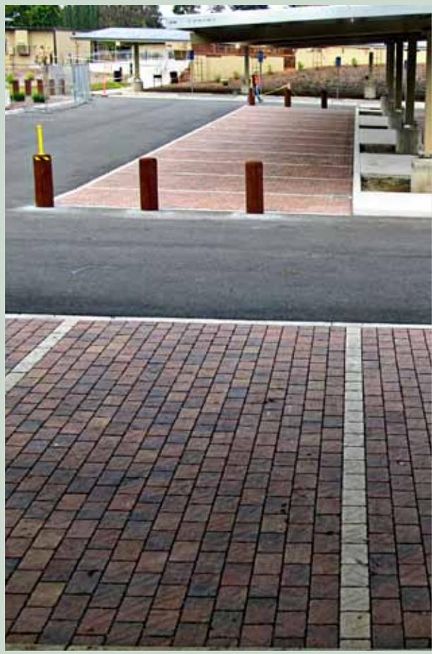
a concern. The joint material is readily available and the strong interlock of the small angular joint aggregate, locks tightly in place, reducing the amount of loose aggregate particles picked up during vacuuming. It's an easy process to rechip any joint areas.
