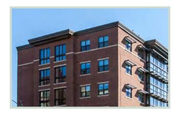
CM suggested we relook at a masonry bearing wall option. They noted the masonry solution was a 'known system that gave peace of mind'. For acoustics, floors and walls were insulated with batt, and a layer of 1/2" plywood was added above cementitious board, separated with a layer of acoustic adhesive. Acoustic adhesive was also added between two layers of gypsum wallboard hung from floor joists.
