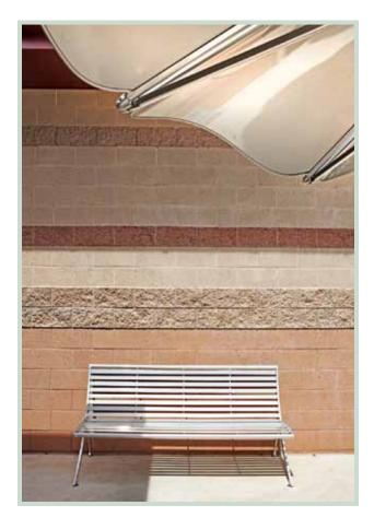
interior temperature, resulting in less heating and cooling of the building. Concrete masonry blocks are very durable and have a low life cycle cost. CMU walls are virtually maintenance free and do not require painting or chemical treatments and their finish qualities including color, texture, and configuration, promote efficient use of resources.
