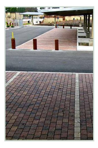
a concern. The joint material is readily available and the strong interlock of the small angular joint aggregate, locks tightly in place, reducing the amount of lose aggregate particles picked up during vacuuming. It's an easy process to rechip any joint areas.
