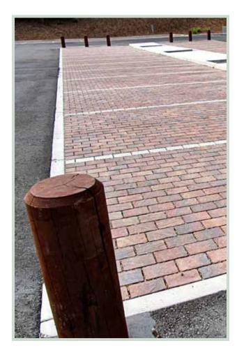
White Quarry Stone permeable pavers were used for the parking stripes. White paint was not wanted on the pavers.
